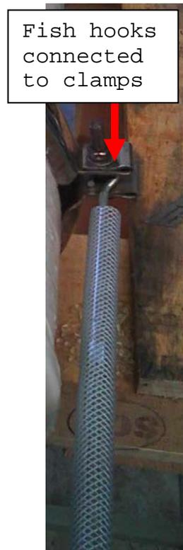
*Figure 3: Fish hook connection points on clamps.*
