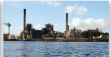
Industrial process water treatment
