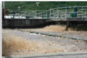
Municipal wastewater treatment
