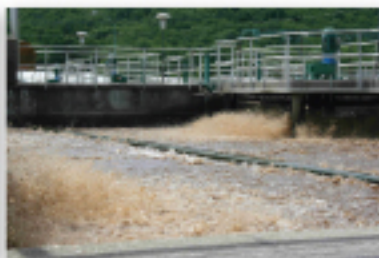
Municipal wastewater treatment
