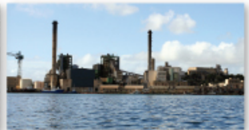
Industrial process water treatment
