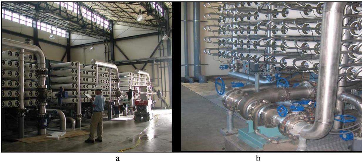
**Figure 1:** Oxnard's (a) 3 RO Trains and (b) Energy Recovery Device (ERD)
