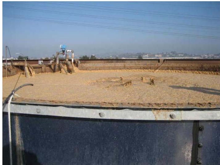
**Figure 6. Top of Aeration Tank during Foaming Event**
