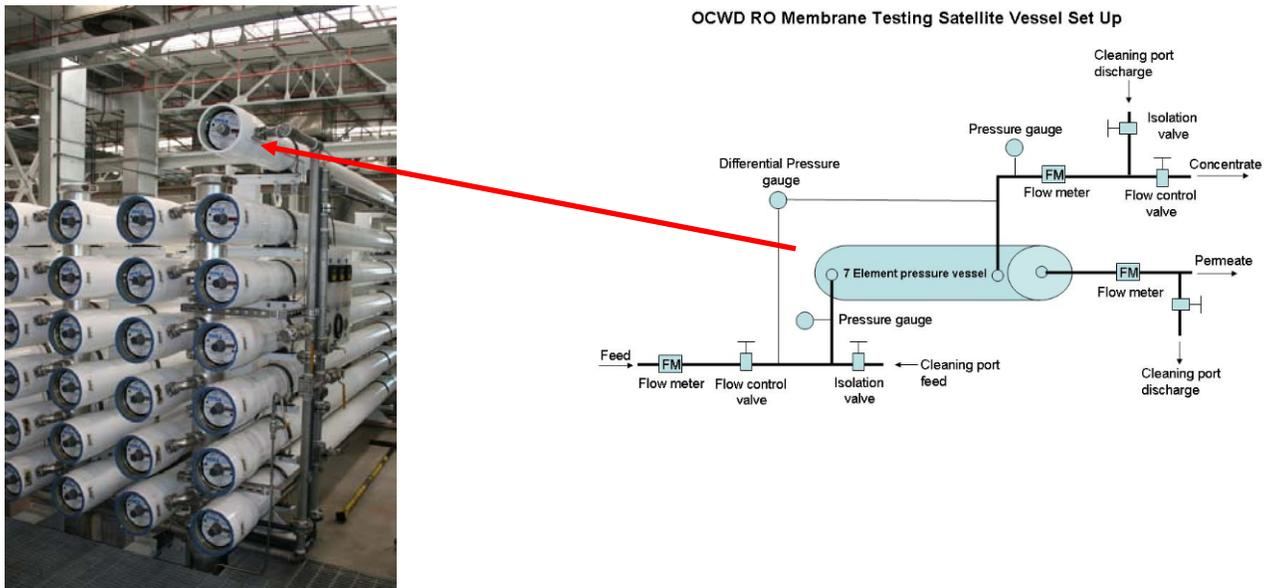
**Figure 1.** Configuration of the test pressure vessel attached to first stage of full scale Train C01.
