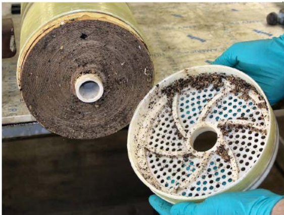
Figure 3. Debris trapped between the seal carrier and the feed end of the lead element.
