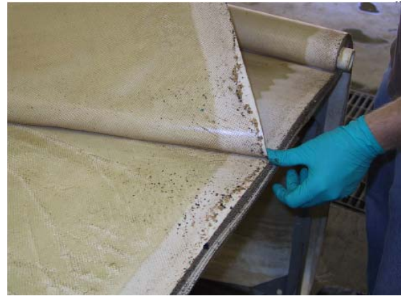
Figure 4. Debris trapped between the leaves of the lead element.
