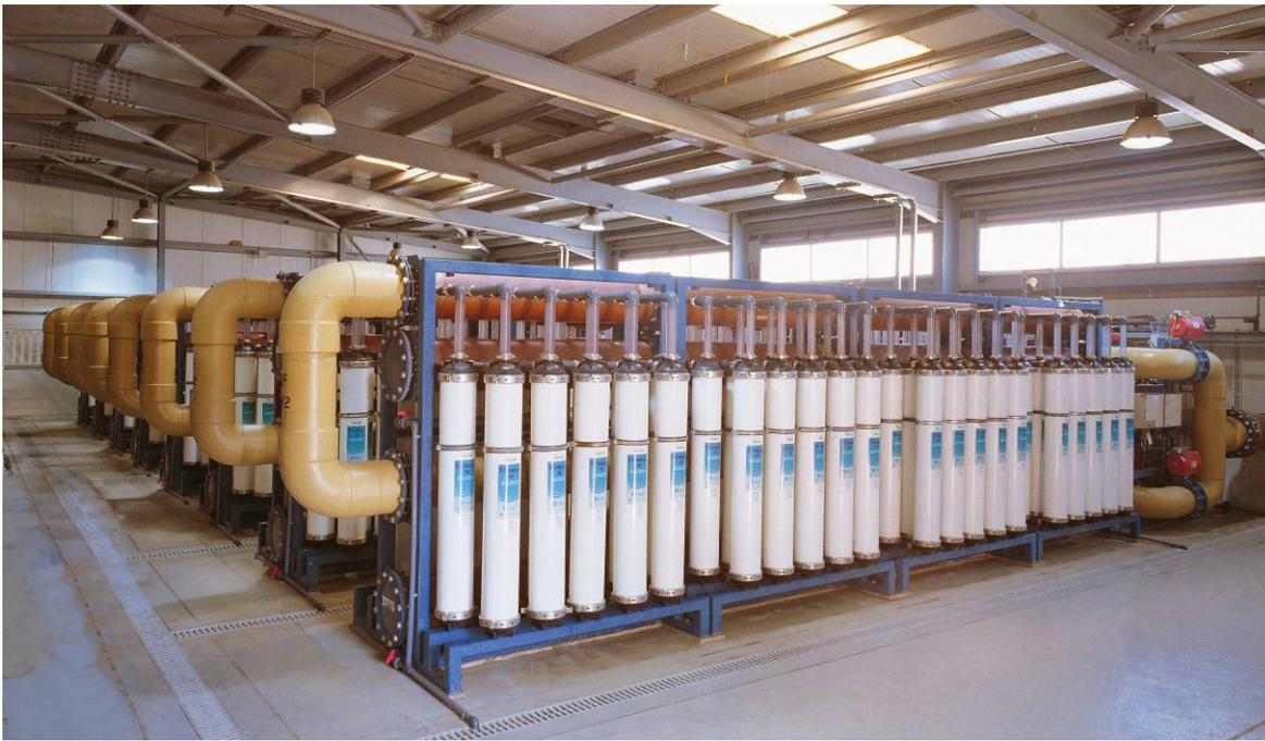
*Picture 7: UF Racks - typical configuration
