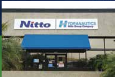
Hydranautics, Oceanside – USA
