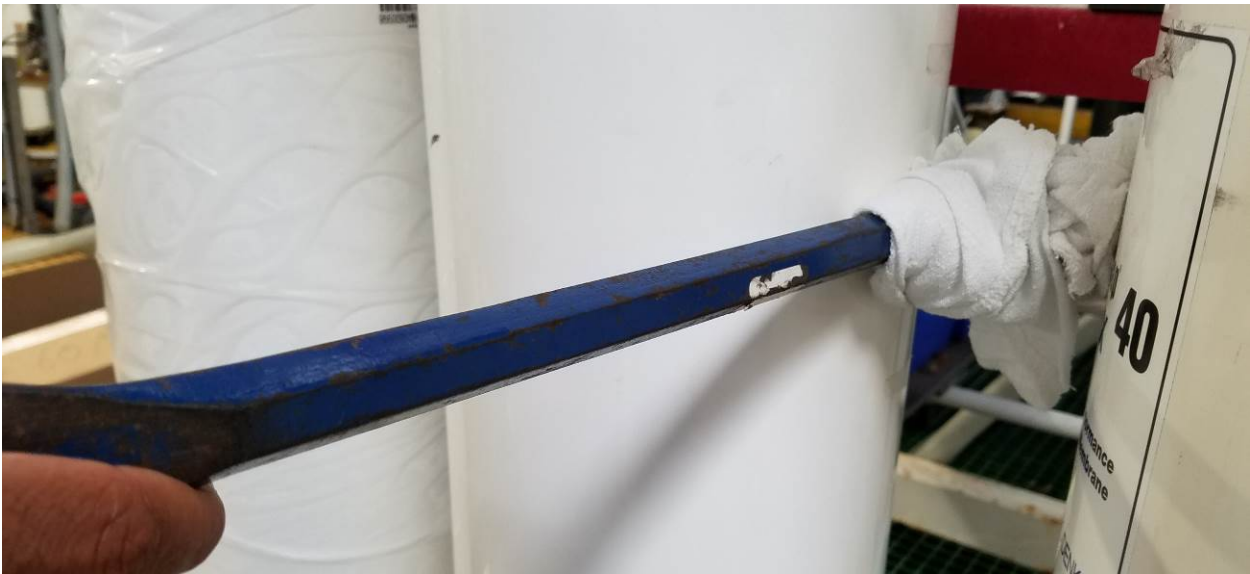
Figure 3: Crowbar with padding to separate modules.
