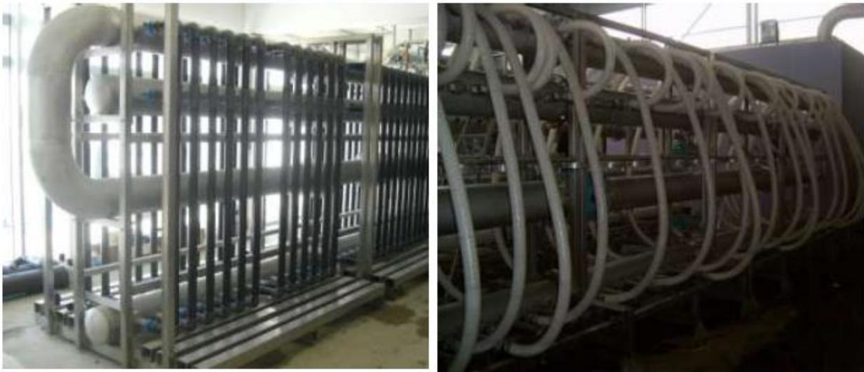
***Figure 1: Examples of rigid and flexible piping used for commissioning phase 1.***
