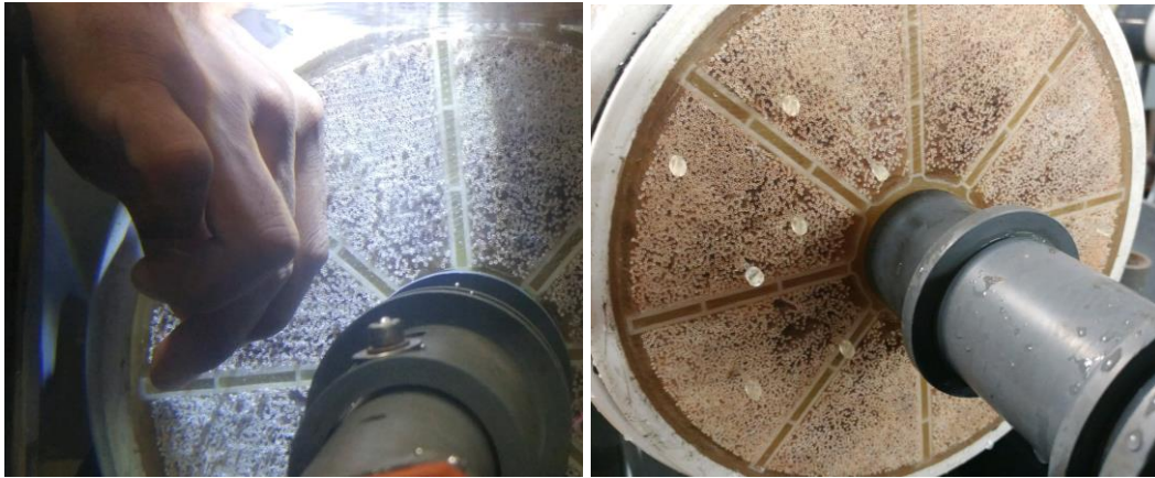
Figure 5: Temporarily installing pins into broken hollow fibers.
