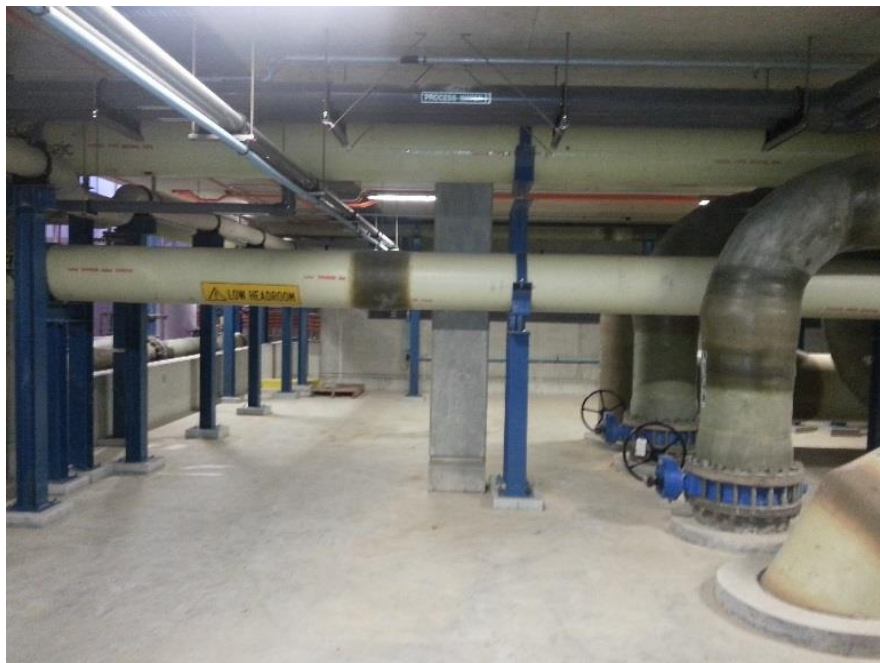
Photo 3 - Adelaide CIP line before modification (courtesy of Acciona)
