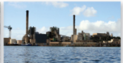
Industrial process water treatment
