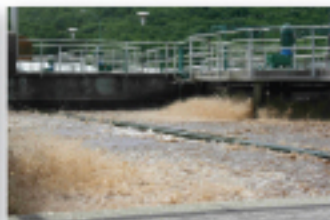
Municipal wastewater treatment
