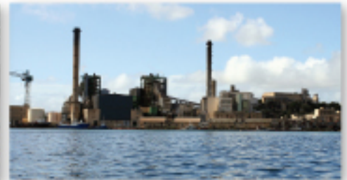
Industrial process water treatment
